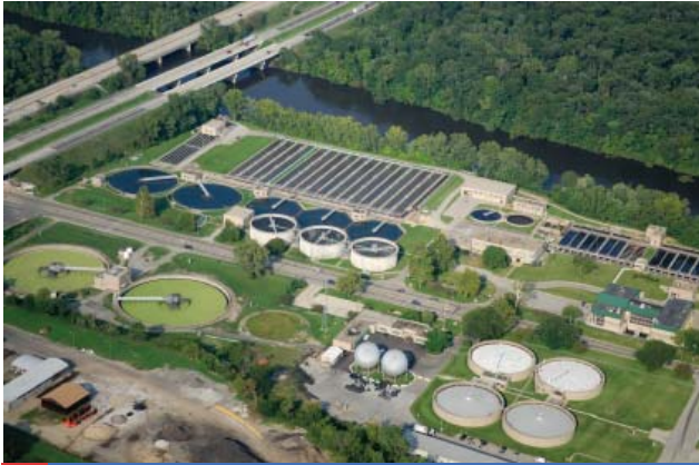
1 Water Treatment Plant
