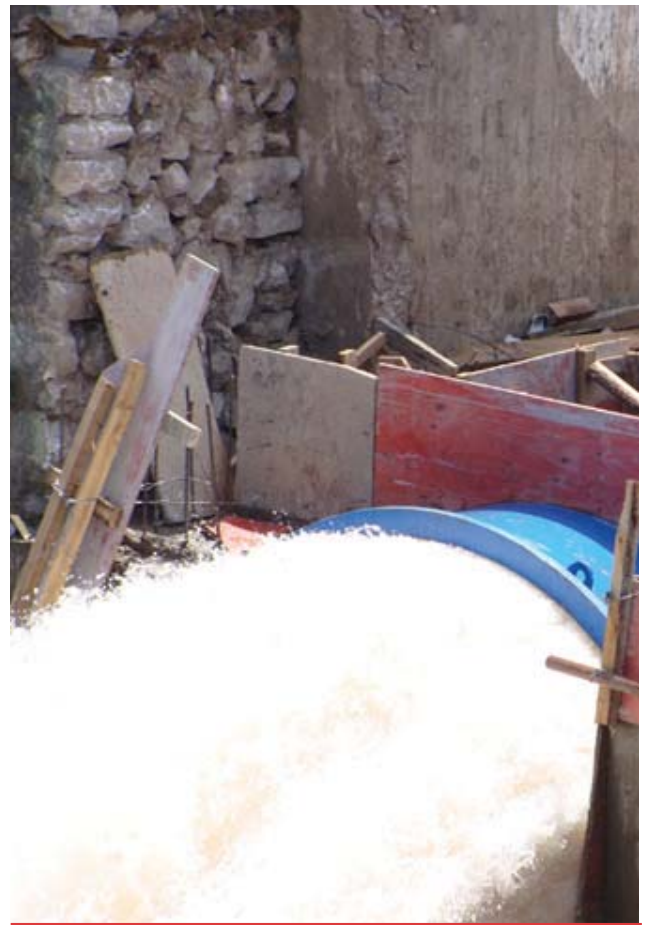
Optional hood discharges flow into confined areas
