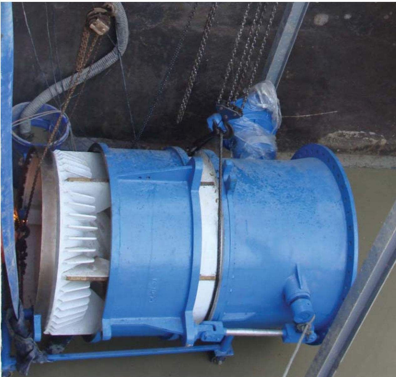
Installation of our DN1400 Fixed Cone Valve
